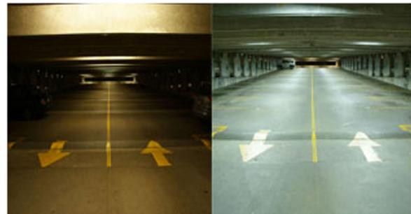
Parking station fluorescent lights (left) replaced by LEDs — increased visibility, decreased energy and maintenance costs<sup>4</sup>.
